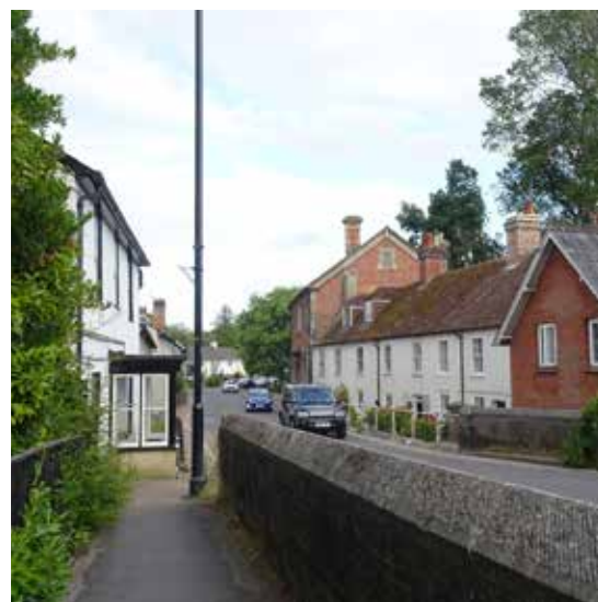
The footway alongside the road bridge © FERIA Urbanism
